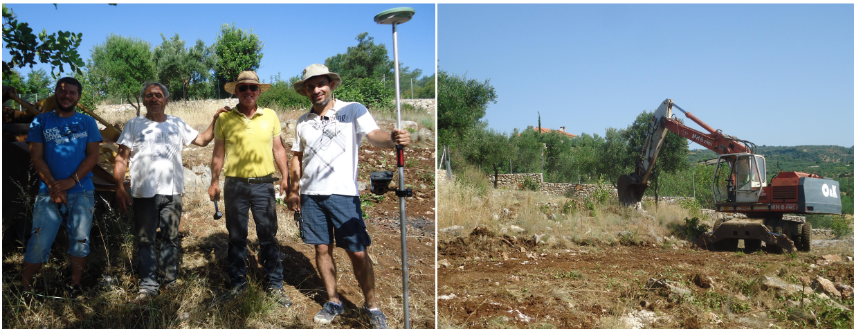
Three excavators and a civil engineer: The beginning of Day One
