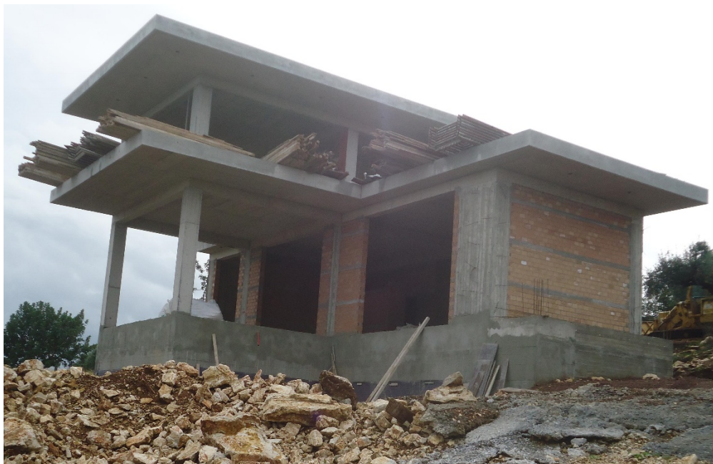
Northern view of the construction so far.
