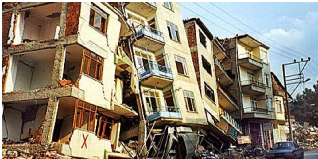
A five-story building containing 17 apartments on the Kalamata waterfront collapsed after the earthquake of 13 th September 1986
